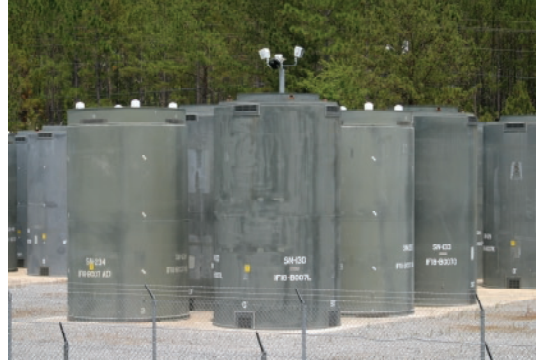
Dry storage at Plant Hatch
