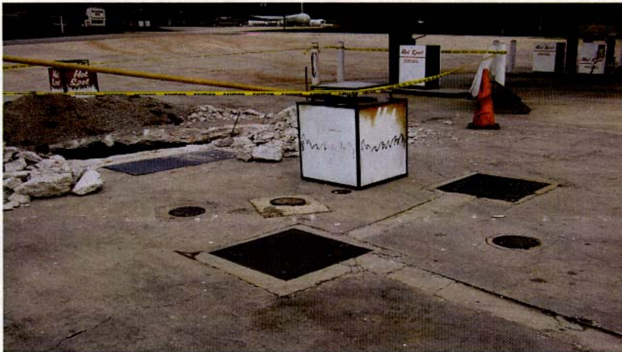
Photo 2. View of excavation north of diesel fuel dispenser island.
