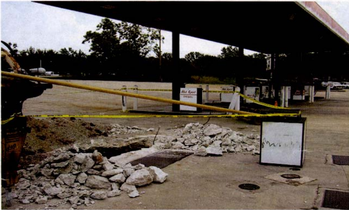
Photo 1. View of excavation north of diesel fuel dispenser island.
