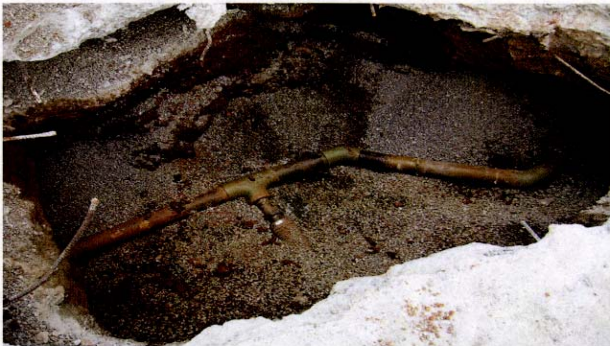
Photo 4. View within excavation north of diesel fuel dispenser island.
