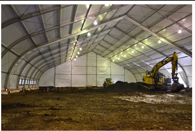
Example Typical Sprung Structure
