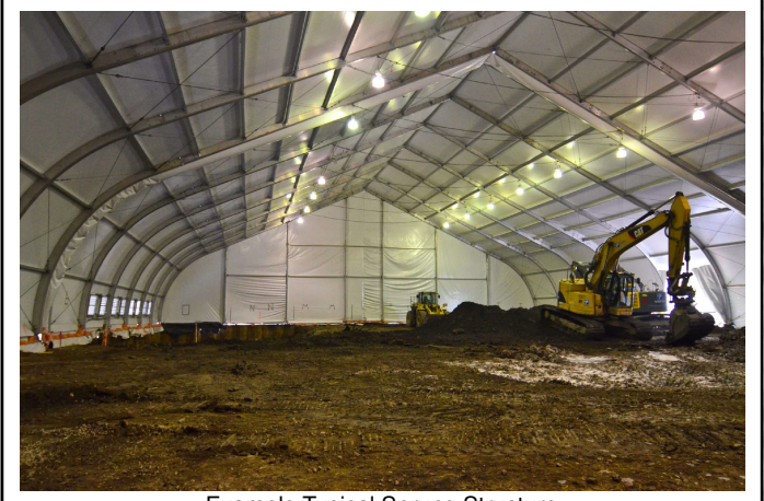
Example Typical Sprung Structure
