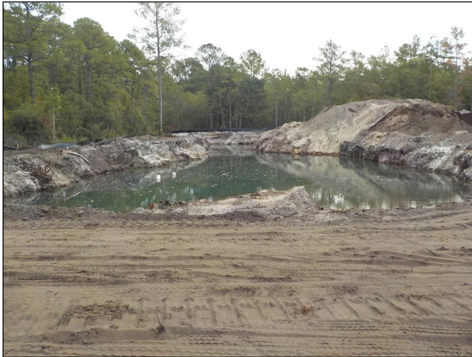
Figure 4. Disturbed area, facing east.
