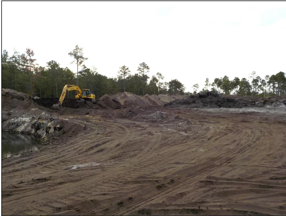
Figure 3. Disturbed area, facing south.
