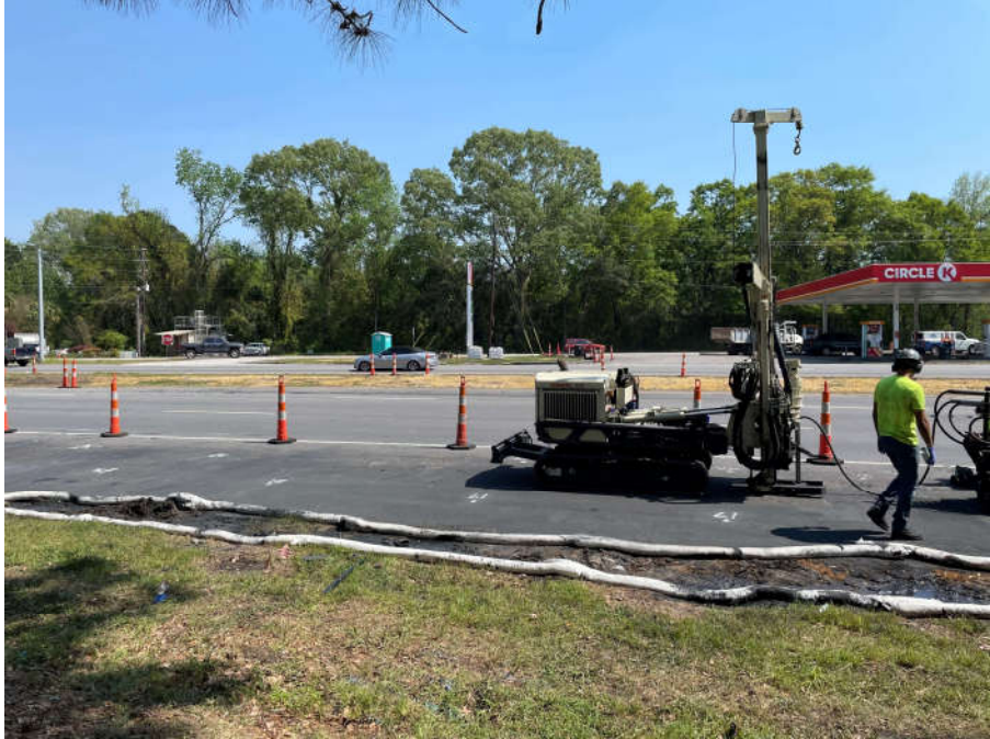
Photo 19: Performing injections in area F 4/7/21
