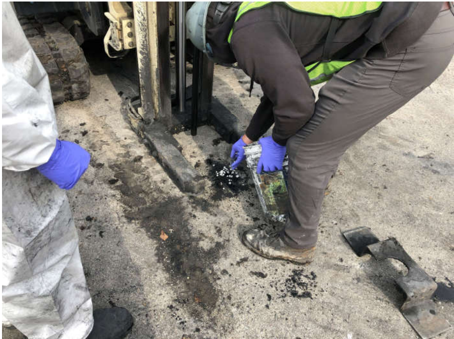
Photo 12: Abandoning injection point with bentonite chips 3/6/21
