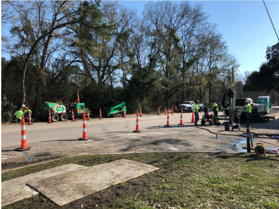
Photo 8: Injecting in Area D while utility clearance continues near MW-15 2/25/21
