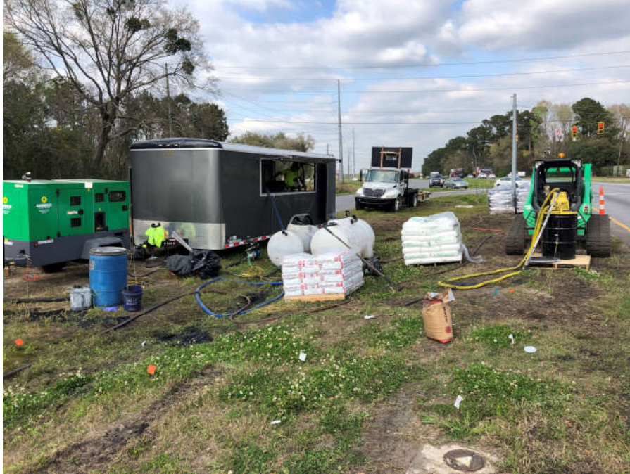
Photo 13: Injection equipment and materials set up for injections in median 3/23/21
