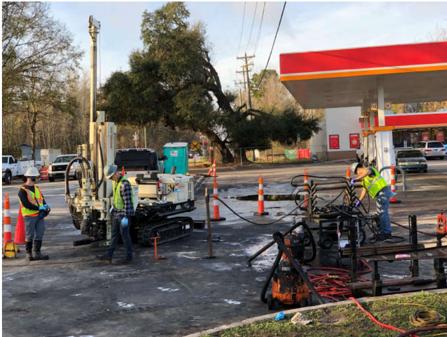
Photo 10: Preparing to pull second tooling string, note plug packer in MW-2 3/1/21
