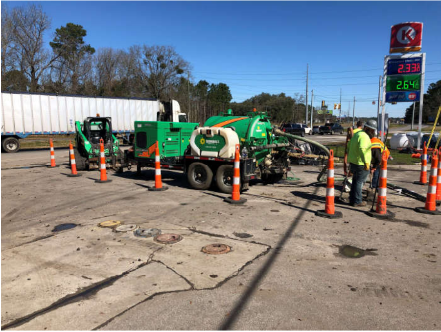
Photo 2: Pre-injection utility clearance 2/23/21
