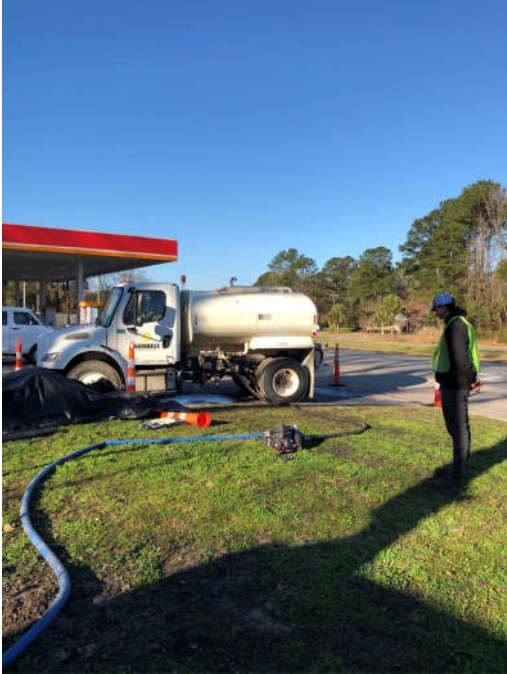
Photo 7: Transferring water from water truck to mixing system 2/24/21
