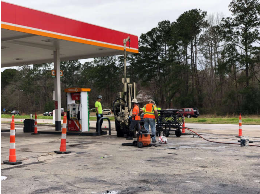
Photo 11: Injecting in area A 3/1/21
