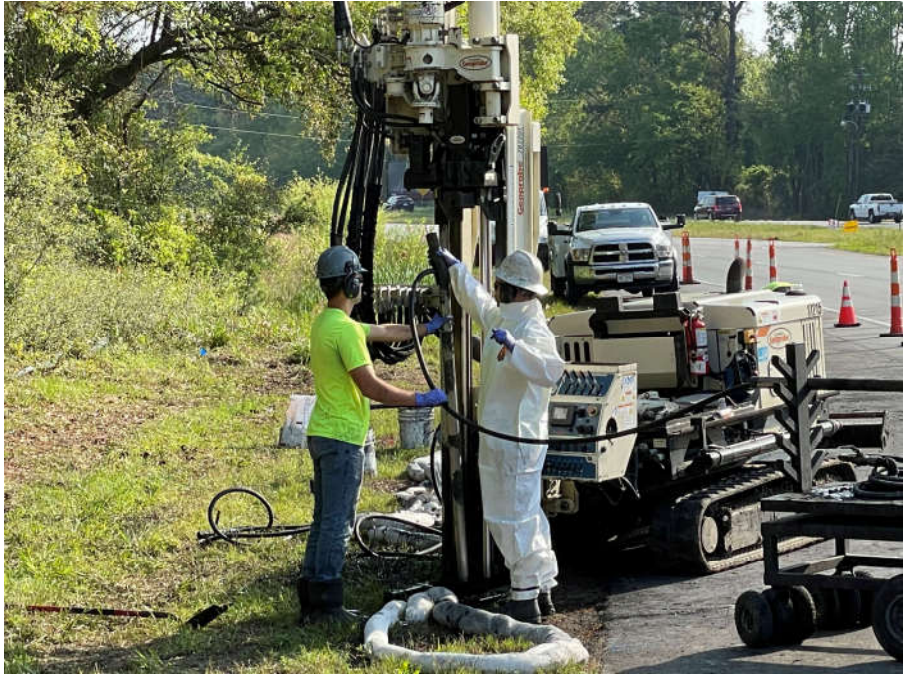
Photo 20: Advancing second tool string in area F 4/8/21
