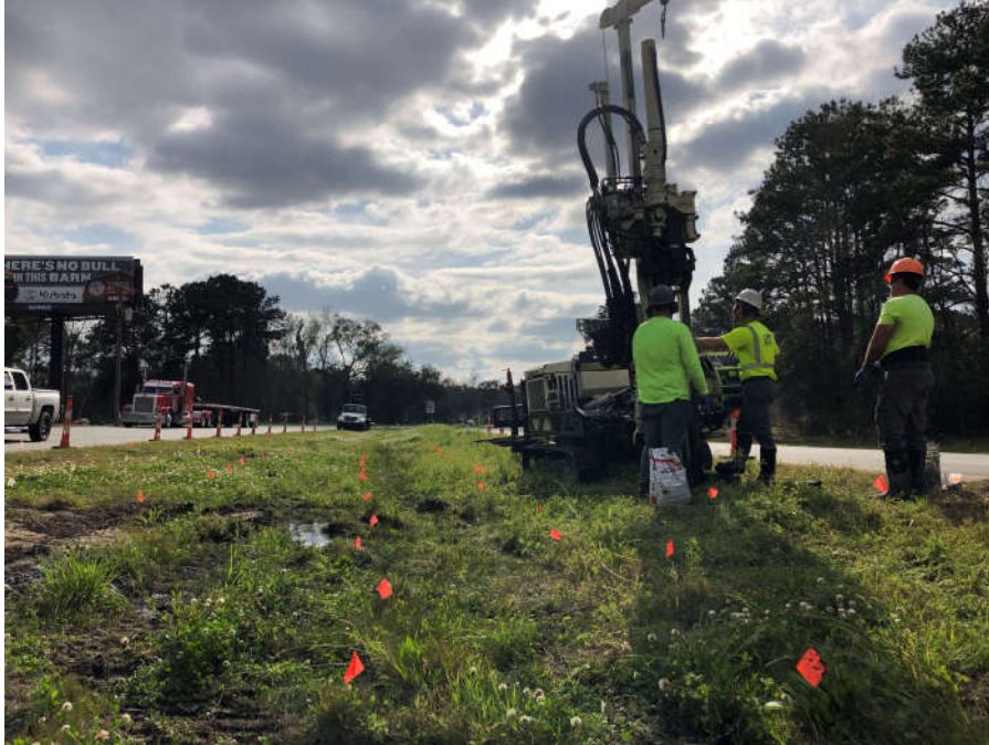
Photo 15: Performing injections in area C 3/23/21
