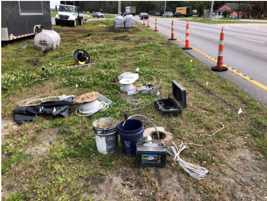
Photo 14: Developing and sampling RW-5 and MW-6 3/23/21
