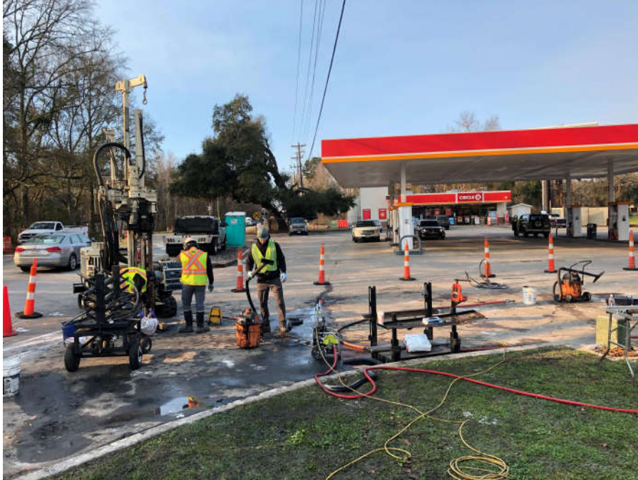
Photo 9: Monitoring MW-2 water level immediately following injections nearby 2/25/21
