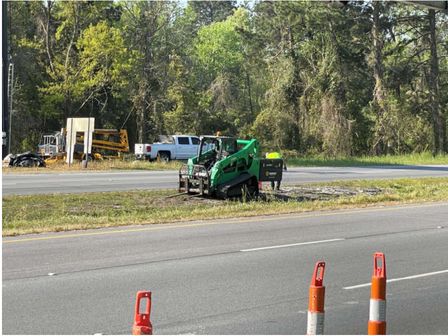
Photo 18: Redeveloping and sampling MW-7 4/7/21
