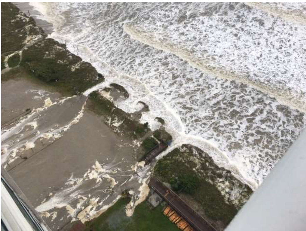
Figure 11. Example of storm surge entering the residential community through dune access paths. Photo taken during the passage of Hurricane Matthew in North Myrtle Beach, SC on October 8, 2016.
