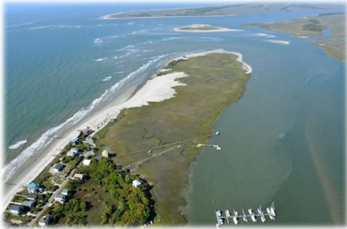
FIGURE 11. EROSIONAL CONDITIONS IN APRIL 2013 PRIOR TO NOURISHMENT AT THE FOLLY BEACH COUNTY PARK.
