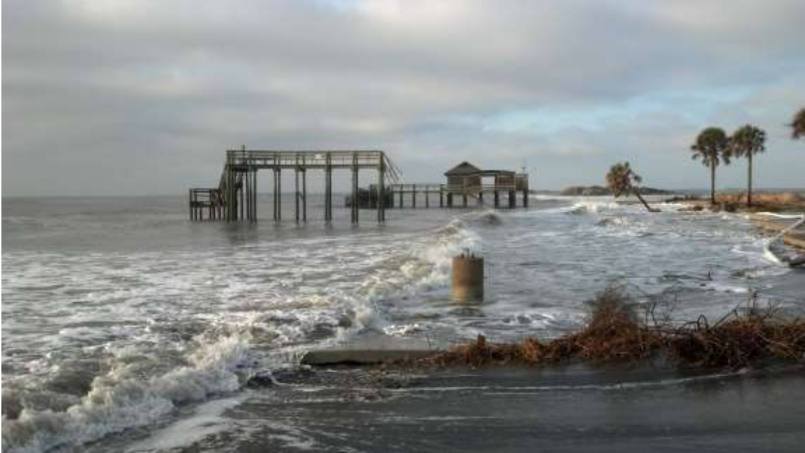
FIGURE 40. FOLLY BEACH COUNTY PARK AFTER HURRICANE SANDY IN DECEMBER 2012.
