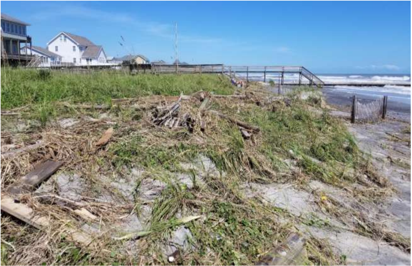
Figure 6. Photo of sand fencing and walkover materials that were destroyed during the passage of Hurricane Irma, increasing the post-storm clean up effort. Photo taken on September 12, 2017 near 10th St. W, looking NE.
