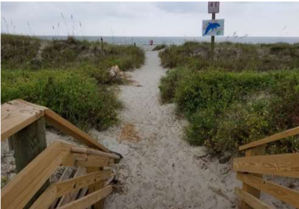
Figure 14. Photo of a public dune walkover that stops short of the seaward toe of vegetation and does not provide sufficient protection of the primary dune. Photo taken at 4th St. E. looking offshore on September 29, 2017.
