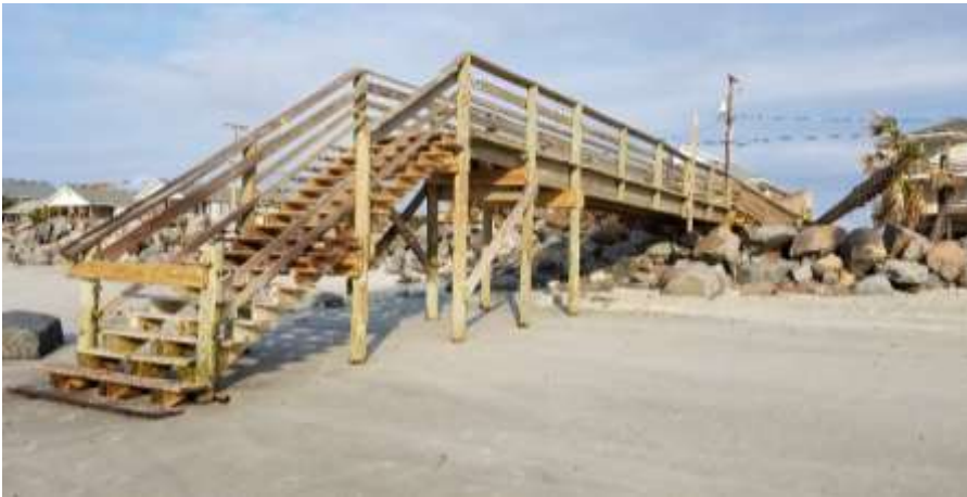
Figure 13. Photo of a dune walkover constructed during a time of wider dunes at the Washout. This walkover has since been retreated. Photo taken on September 30, 2017 looking onshore.
