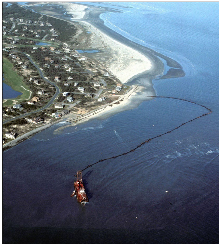
FIGURE T-9. [UPPER] 1989 plan for realignment of the northern channel and nourishment south of Renken Point. [LOWER] Start of dredging operations in February 1990 at Renken Point.
