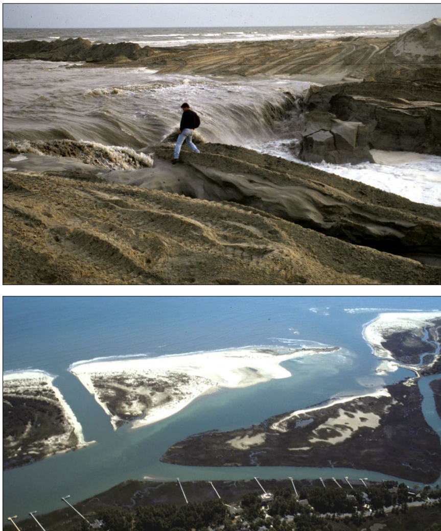
FIGURE T-10. The second relocation of Captain Sams Inlet in April 1996. [UPPER] First tide into the channel basin on 4 April during a rising tide. [LOWER] The new channel (left side) before completion of the closure dike across the old channel.
