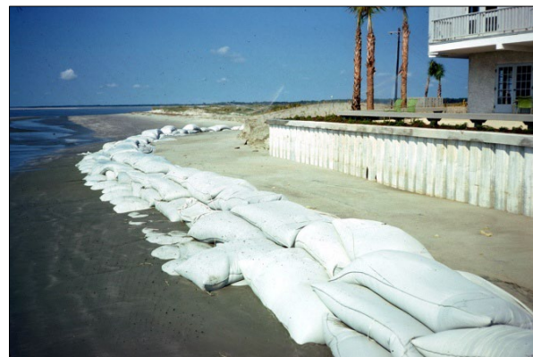
FIGURE T-4. Shore-protection structures at the Beach Club in September 1974 prior to the club's opening.
