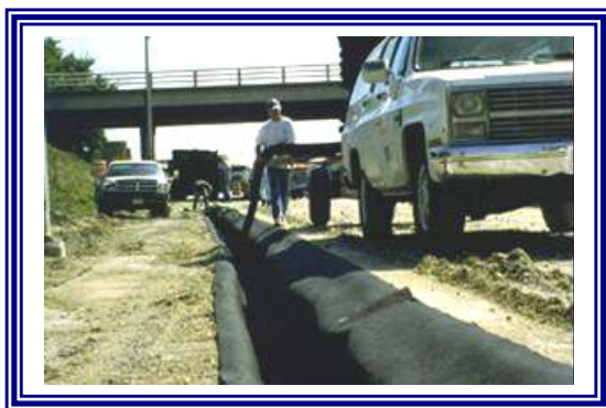
Subsurface Drain
