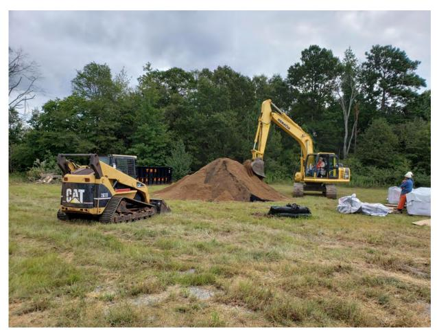
Photograph 6: Mixing sand and carbon at stockpile area.
