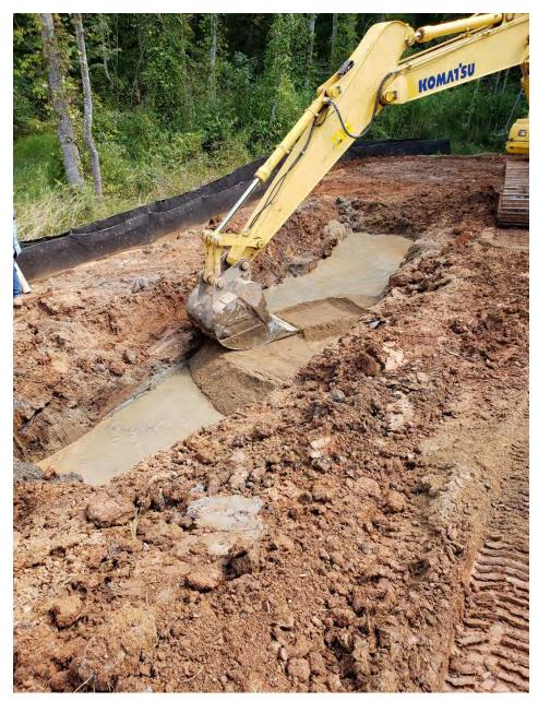
Photograph 8: Compacting backfill with excavator.
