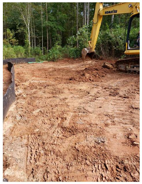
Photograph 9: Covering south end of backfilled trench.
