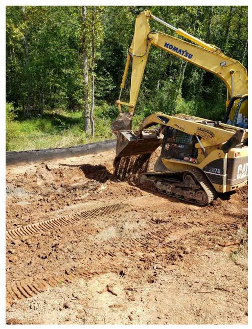
Photograph 7: Backfilling with sand and carbon mix.
