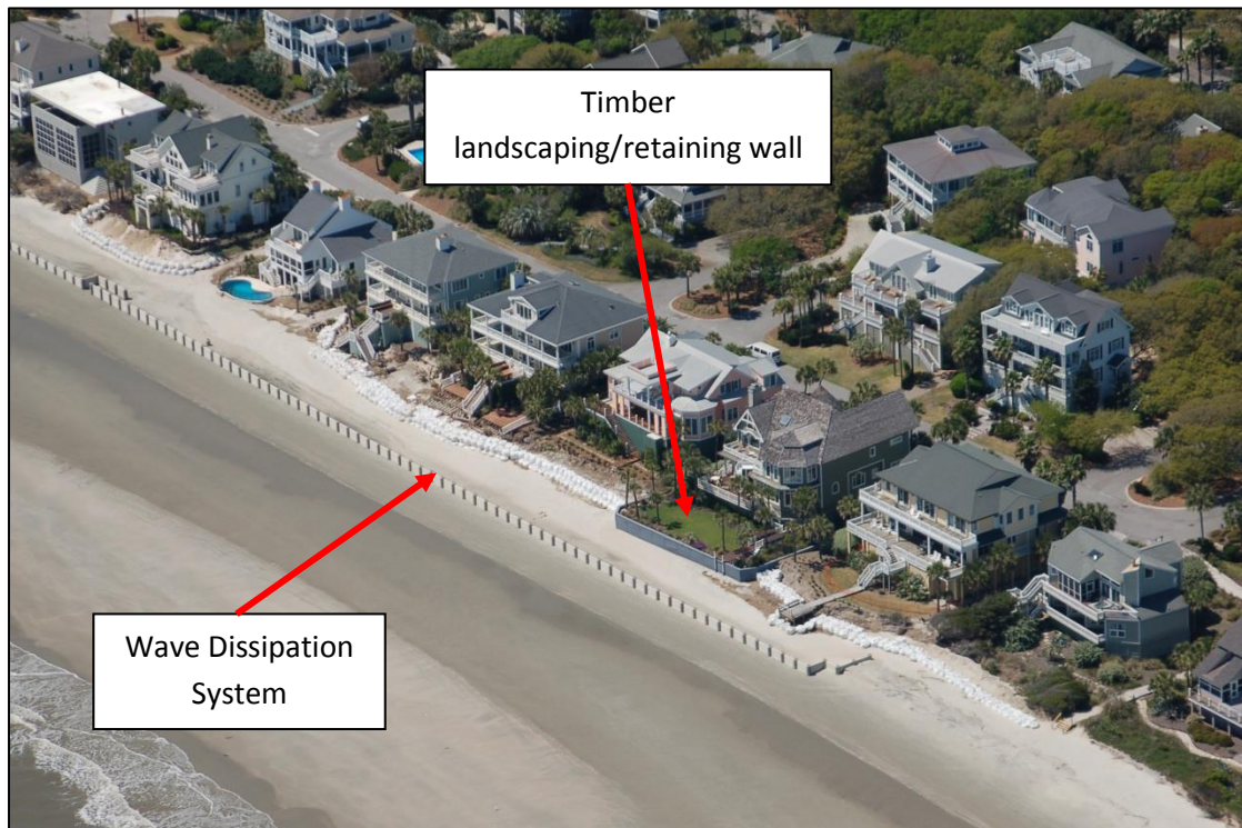
Figure 22. April 5, 2016 photo of Wave Dissipation System installation at Beachwood East (same area as shown in Figure 17). WDS ties into rock revetment at west end, see Figure 21. A timber retaining/landscaping wall is also shown.
