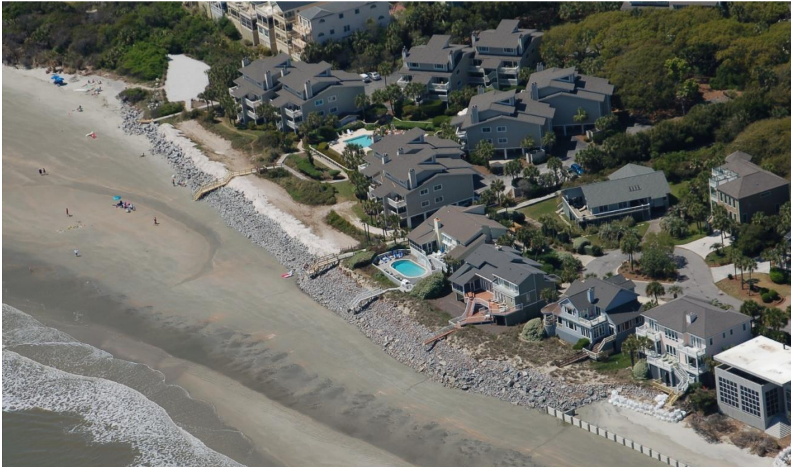
Figure 21. April 5, 2016 photo of exposed rock revetment near Seagrove/Beachwood East.
