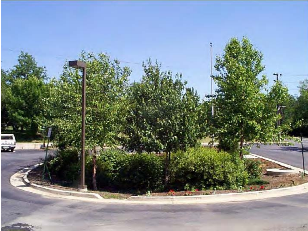
Figure 4-8: Bioretention in a Parking Lot Turnaround
