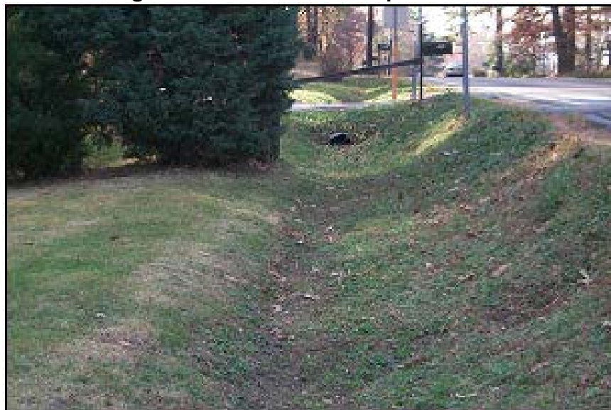
Figure 4-15: Grass-Lined Open Channel
