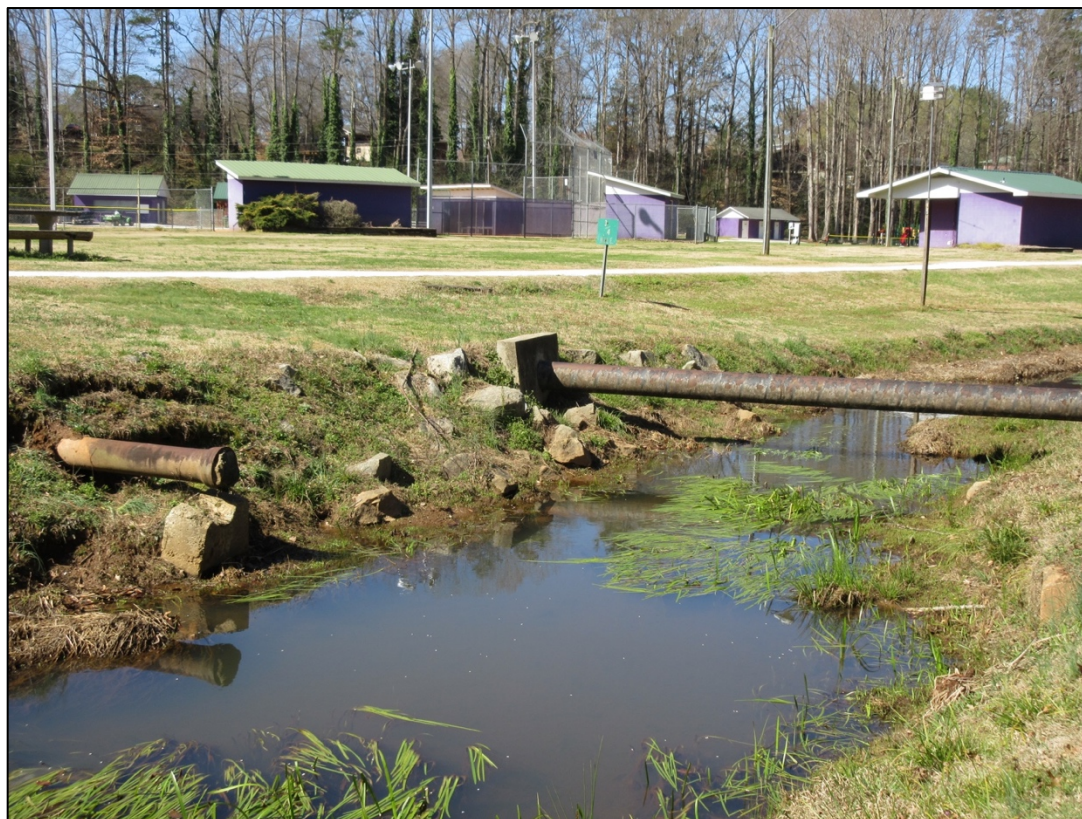
Fig.18. Previously sealed and replacement sewer lines hover just a few feet over unnamed tributary leading to Cane Creek, which runs through Sertoma Field, Walhalla, SC.
