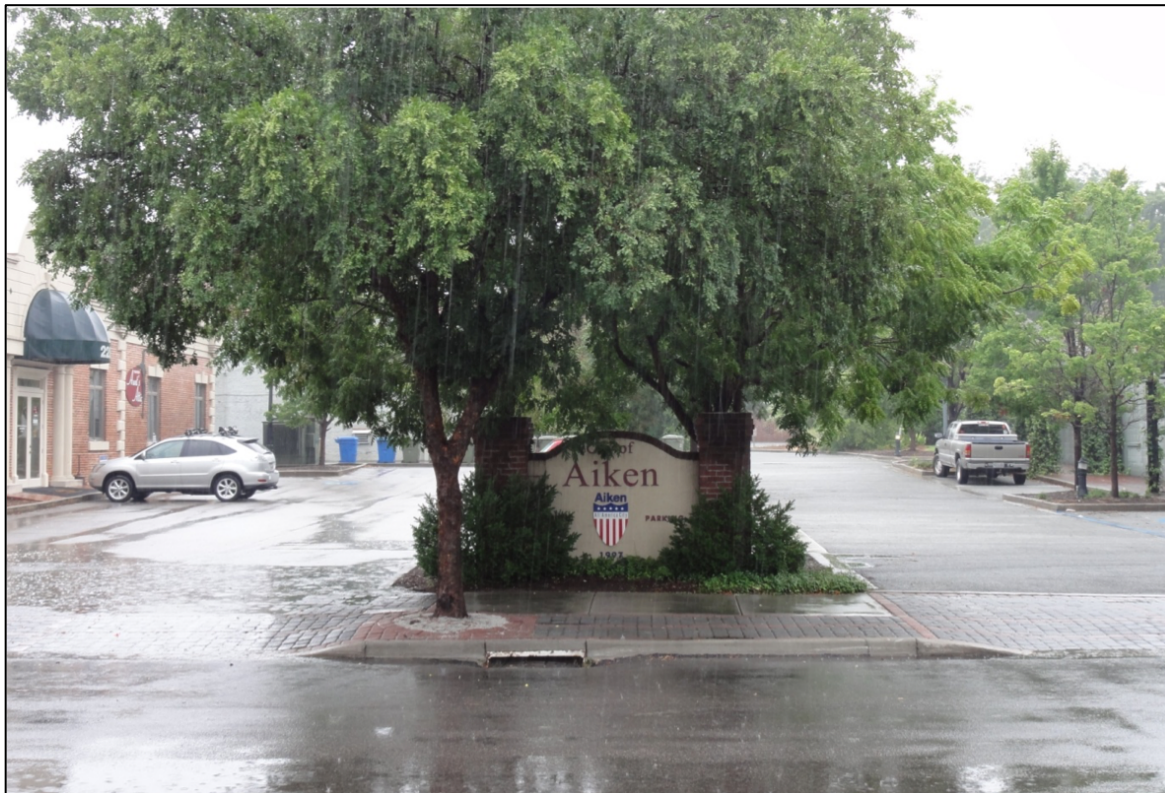
Fig. 28. This image from Aiken, SC demonstrates the ability of a porous asphalt road (right) to quickly infiltrate rain water, in comparison to standard asphalt (left) showing puddles (Source: Calvin Sawyer, Ph.D., Clemson University).
