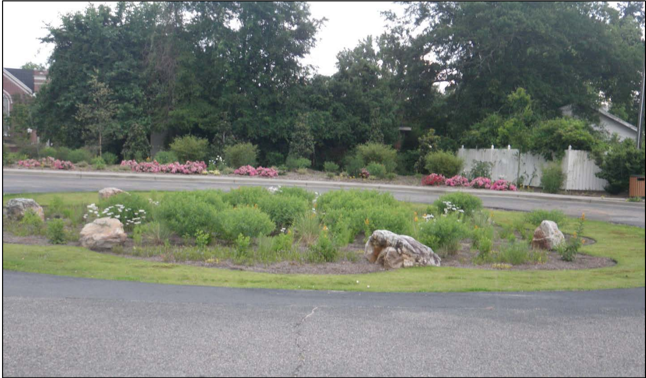
Figure 5-5: Bioretention at Ronald E. McNair Memorial Park, Lake City, SC
