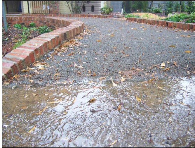
Example of pervious pavement at the Upstate Forever office in Greenville, SC (above).
