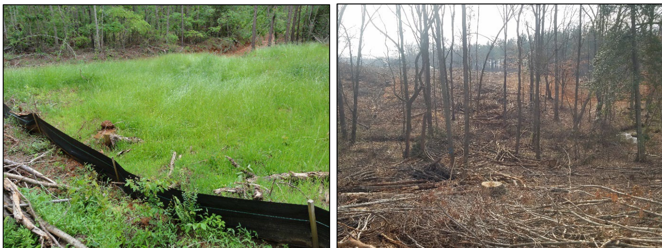
Examples of BMPs during timber harvests; grass and silt fence (left), debris stabilization (right). Source: SCFC.
