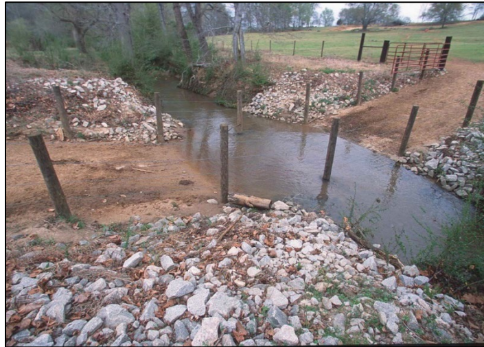
Example of Armored Streambank Crossing (above).
