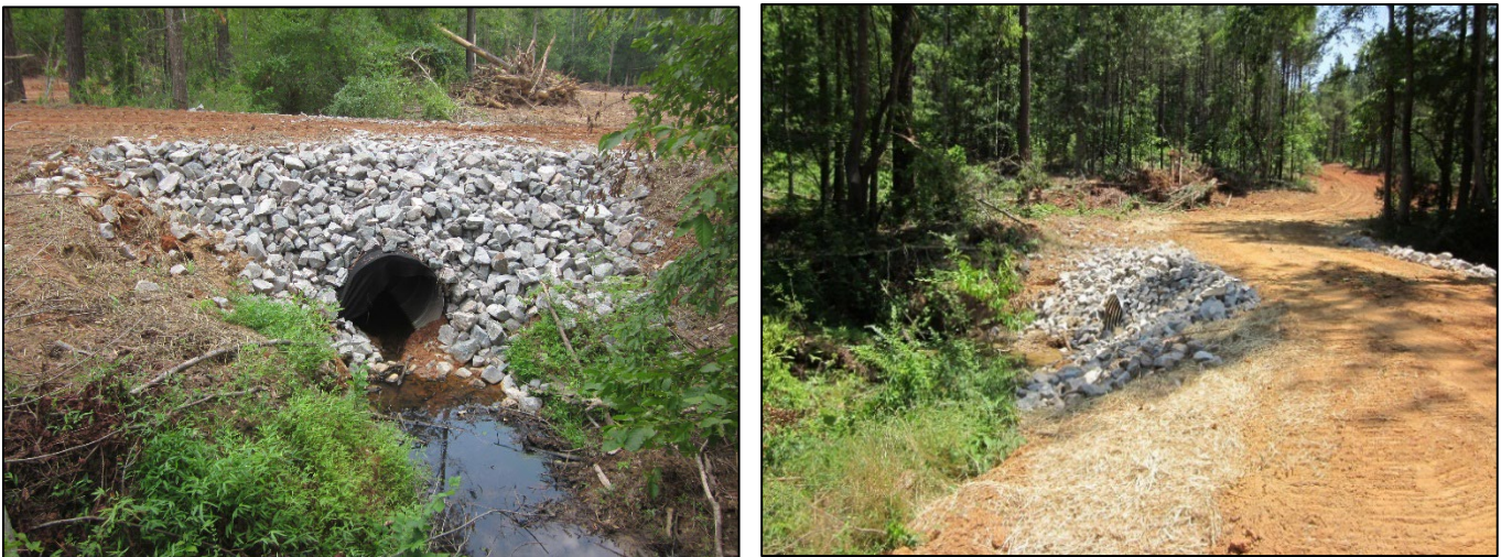
Examples of stabilized culverts (above). Source: SCFC.
