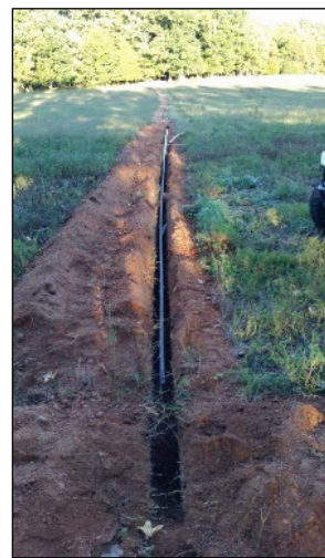
Examples of alternative watering source installed (left) and linear pipeline (right) in the Walnut Creek watershed.
