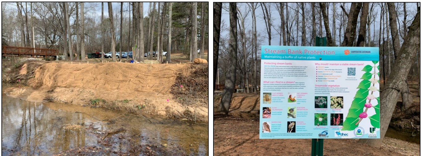
Example of a riparian buffer stream repair on Brushy Creek, Greer, SC. Installed erosion control fabric with livestockes (left) and educational signage (right).
