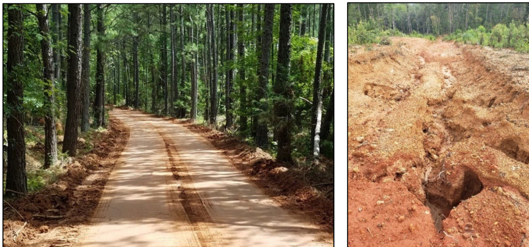
Stabilized dirt forest road (left) and un-stabilized dirt forest road (right). Source: SCFC.
