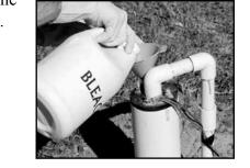
4. After the bleach has been added, run water from an outside hose into the well casing until you smell chlorine coming from
