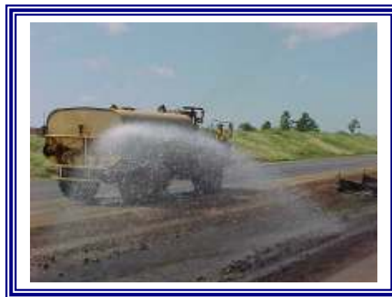
Dust Control by Sprinkling Water
