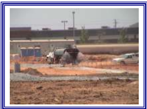
Dust Control by Sprinkling Water
