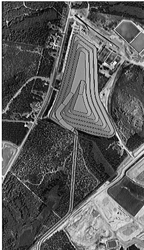
Figure 6: Low-Grade Stockpile at Parking Lot
