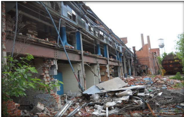
Before VCC Work
