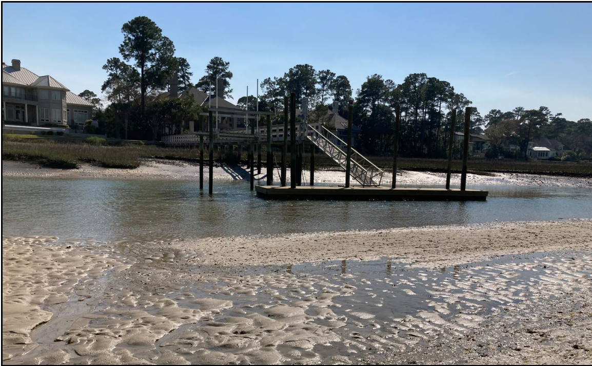
Figure 4. March 2022 drone oblique aerial imagery taken from southern end of Pine Island spit looking SSW across Park Creek inlet toward marsh and houses along Ribaut Dr.
