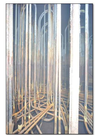
Figure 4.1-5: Type I Tank (Tank 12H) Cooling Coils
